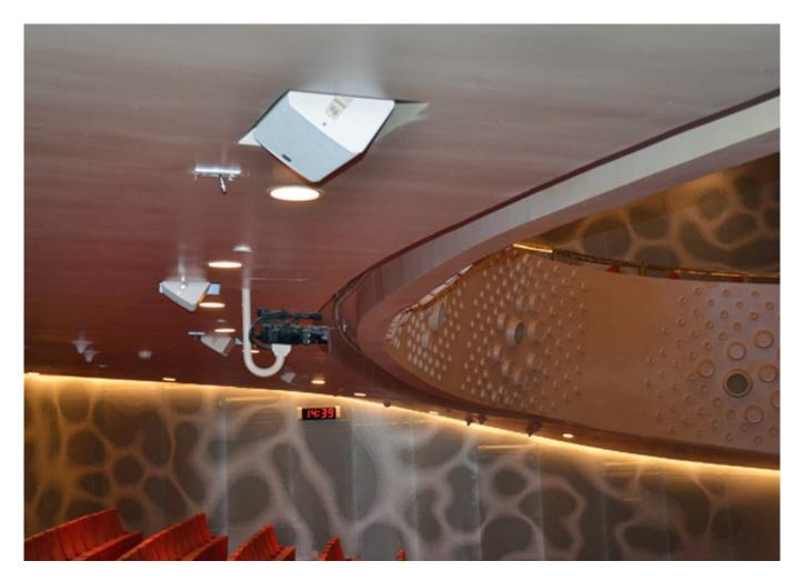
20 x K&F CA 106 units are installed below the balconies to cover the range of sound shadows. 5 x K&F CA 1215 full-range speakers and 3 x K&F SWi 115E subwoofers are hung vertically from the theatre's ceiling to achieve effects such as the voice of God. All speakers in combination form an acoustically perfect 360° hall effect throughout the auditorium, which is almost perceived as the naturally reflected sound.
