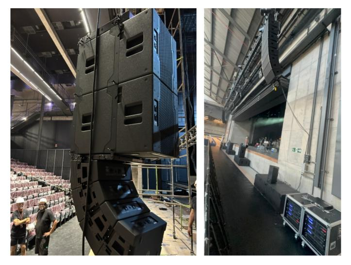
Commenting on the installation, Esteban Risso, Commercial Director of Gobos do Brasil, said: "We achieved extremely linear coverage, with only a 1.5dB variation between the first and last rows. The suspended cardioid subwoofer arrangement eliminated bass spill onto the stage and ensured consistent low-frequency coverage throughout the theatre, without overwhelming audiences in the front rows."
